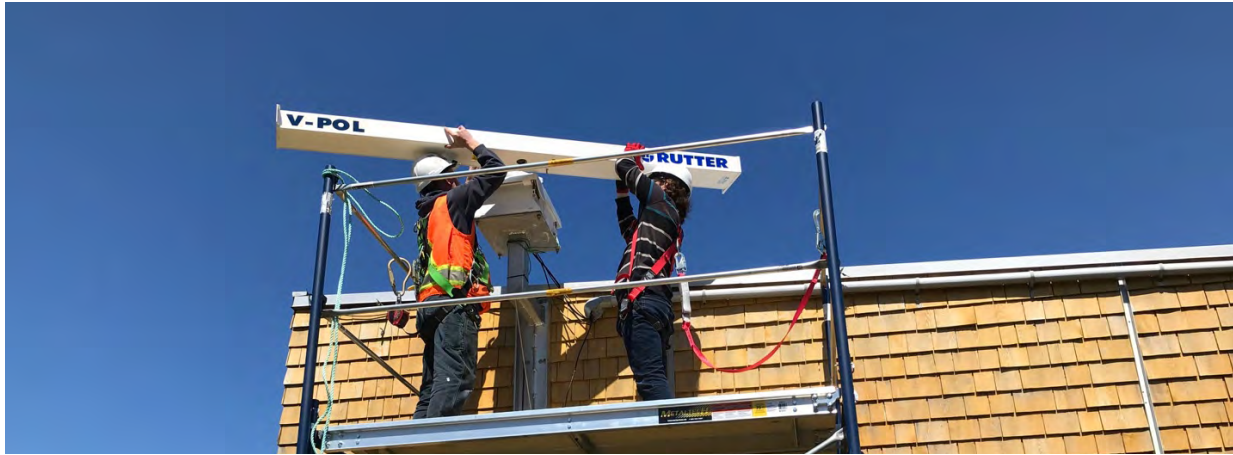
Installing a high-resolution marine radar at the FORCE facility
